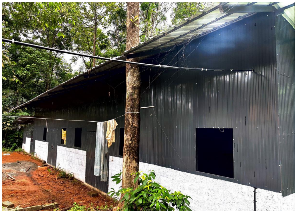
Office rooms and Shelters
